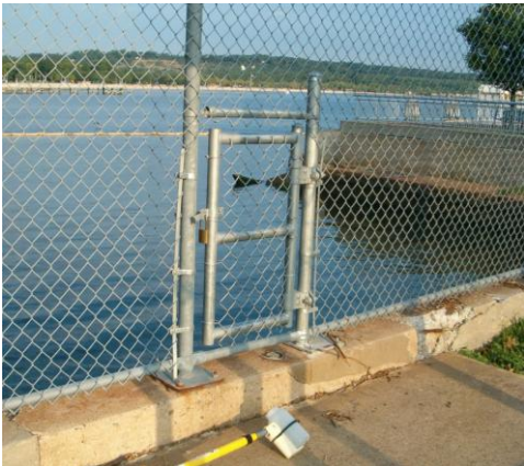
Gate for sampling Powerhouse Drain (photos by Carol DiPaolo, 8/4/10 and 7/19/10)
