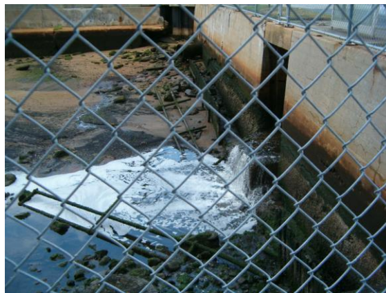
Soap suds flowing from Powerhouse Drain on 7/19/10
